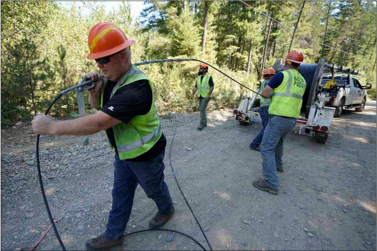
Carl Roath, left, a worker with the Mason County Public Utility District, pulls fiber optic cable off of a spool, as he works with a team to install broadband internet service to homes in a rural area surrounding Lake Christine near Belfair, Washington.
